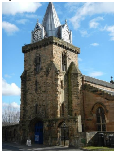
Fig 5. Parish Church of St Peter, West Tower
