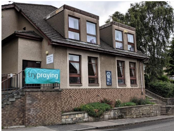
Fig 16. Inverkeithing Baptist Church (Bess Rhodes)
